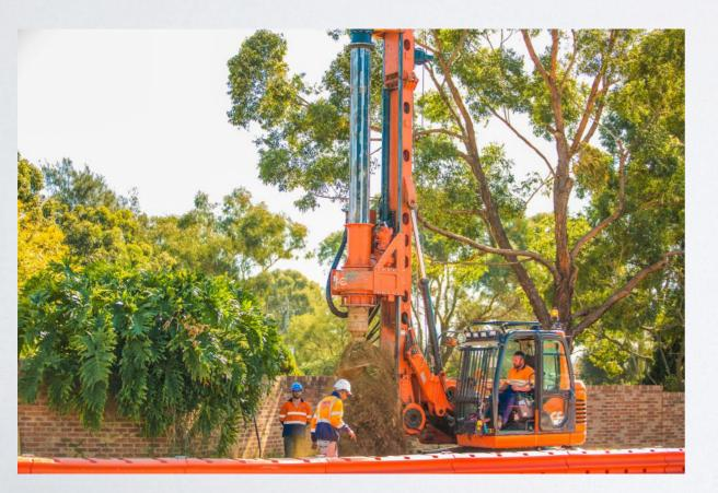
Werrington Client: RMS Scope of works: 400piles dia 750mm & 900mm bored to 6.5m Project status: Intermediate \$750,000 Sector: Civil Application: Noise barrier wall Equipment: CF6 Year: 2016
